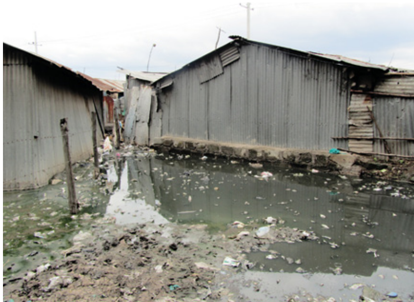
Open drain in Mukuru Slum, Nairobi, Kenya
