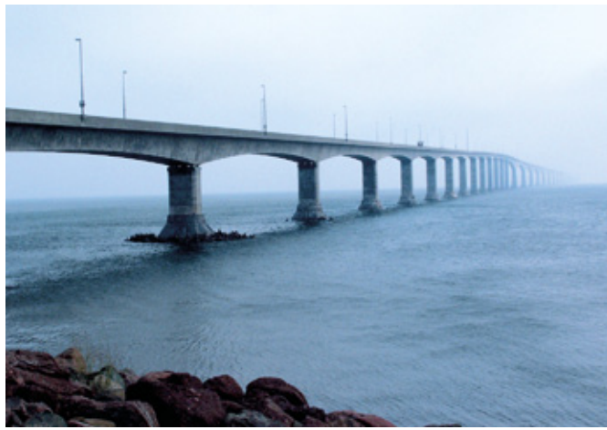
The Confederation Bridge, Canada
